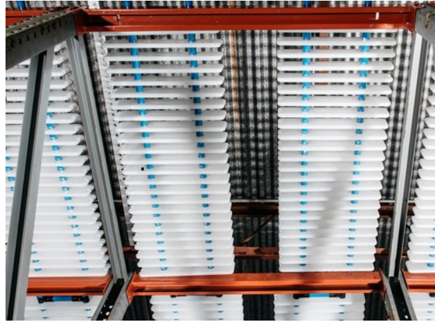
Fig. 10. PCM filled polymer tubes suspended in ceiling [18]
